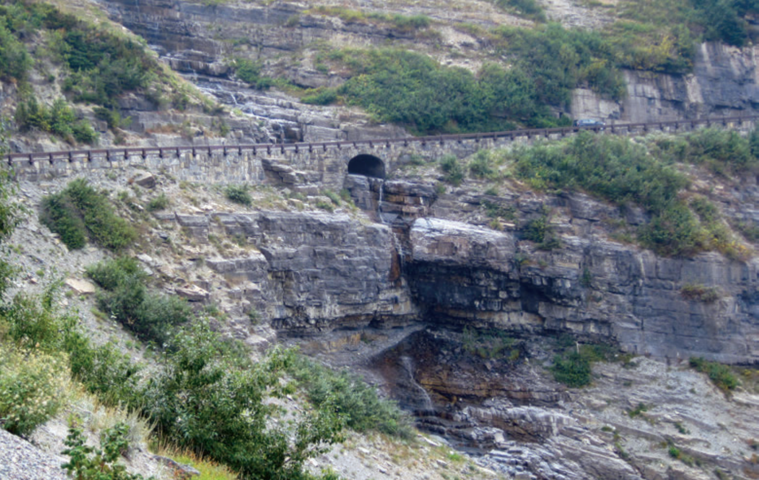
One of the many archways along the Going-to-the-Sun Road which allow the glacier-fed waterfalls to flow, uninterrupted, under the roadway and into the valley rivers below.
