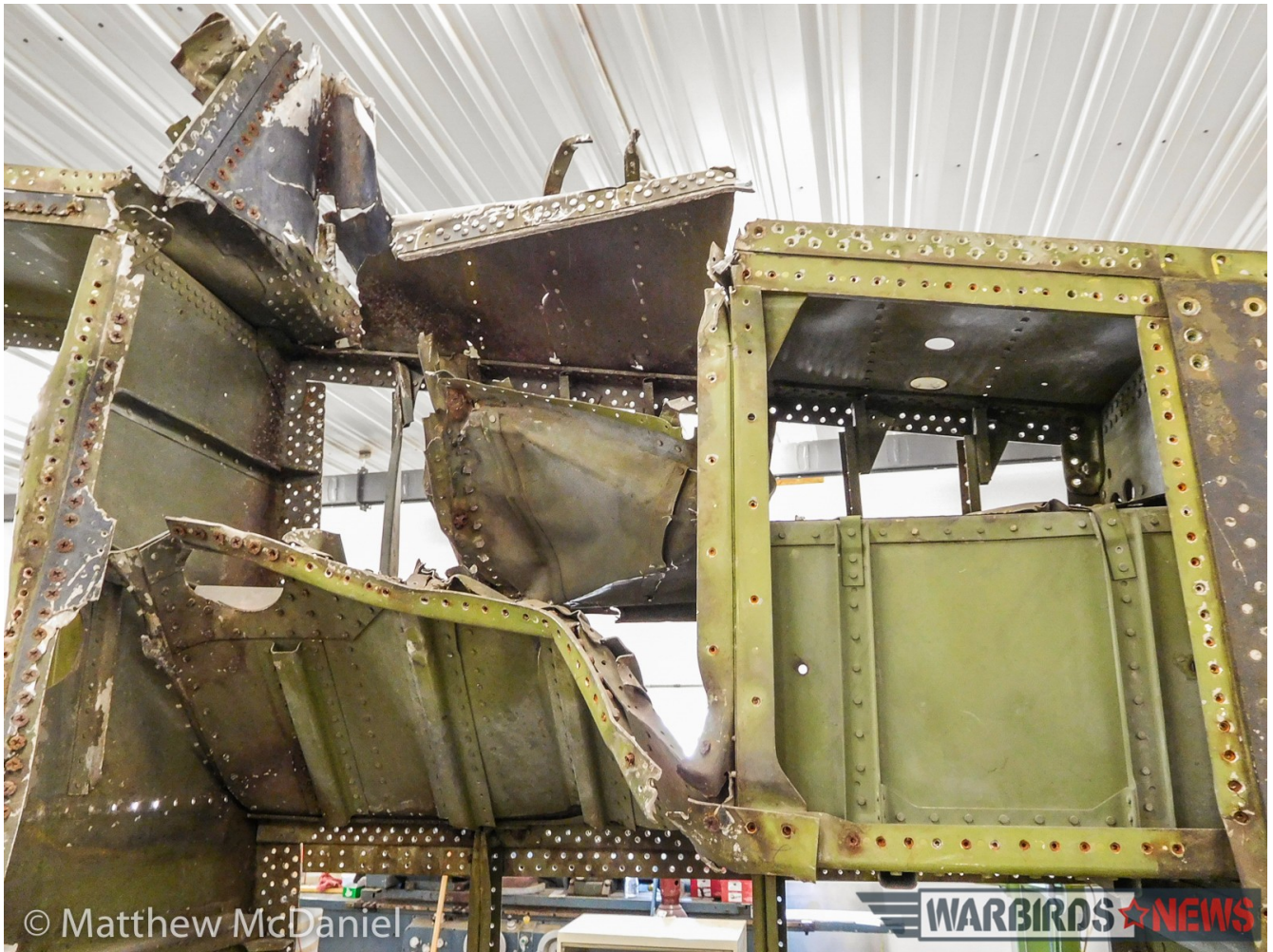
A close-up of one of the most extensively damaged areas of the Helldiver's inboard wing section (photo by Matthew McDaniel).
